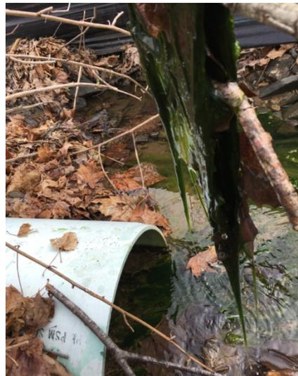
*This outfall is partially submerged and a clean catch of its discharge is not possible. If tidal influences are strong, wait until low tide to sample.*
